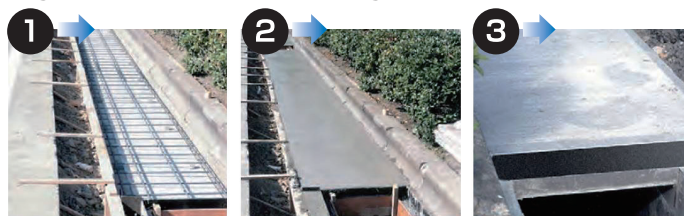
In-ground concrete drain-covers
