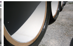
Filling the end face of the sewer pipe with TS seal
