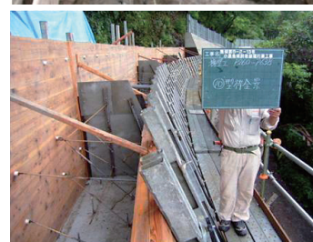
In-ground forms used as a substitute for wooden joint forms
