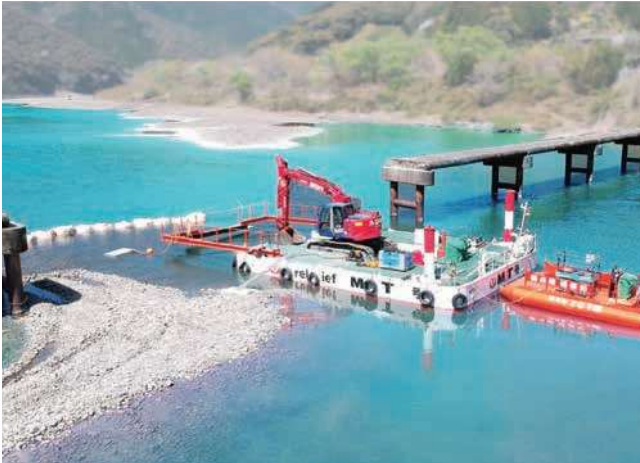
Repair work subsidence bridge at Shimanto River
