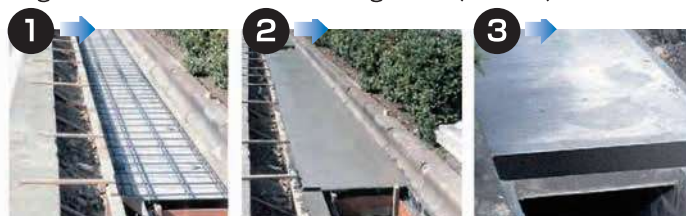
In-ground concrete drain-covers
