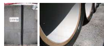
Filling in the joints of a seawall Filling the end face of the sewer pipe with TS seal
