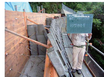
In-ground forms used as a substitute for wooden joint forms
