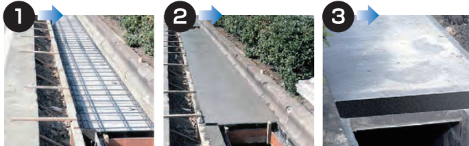
In-ground concrete drain-covers
