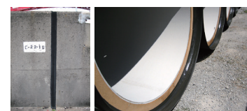
Filling in the joints of a seawall TS seal
