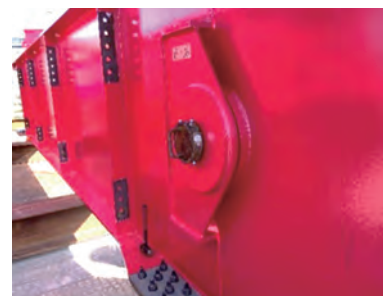
Pin connection structure
